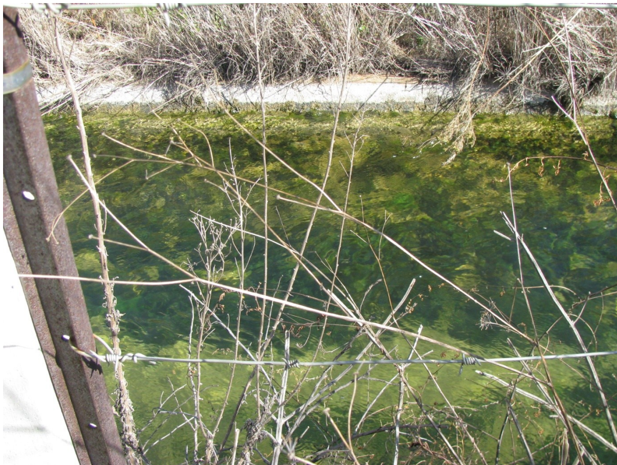
Photo 5.1: Photo of the Schoonspruit canal illustrating build-up of algae
